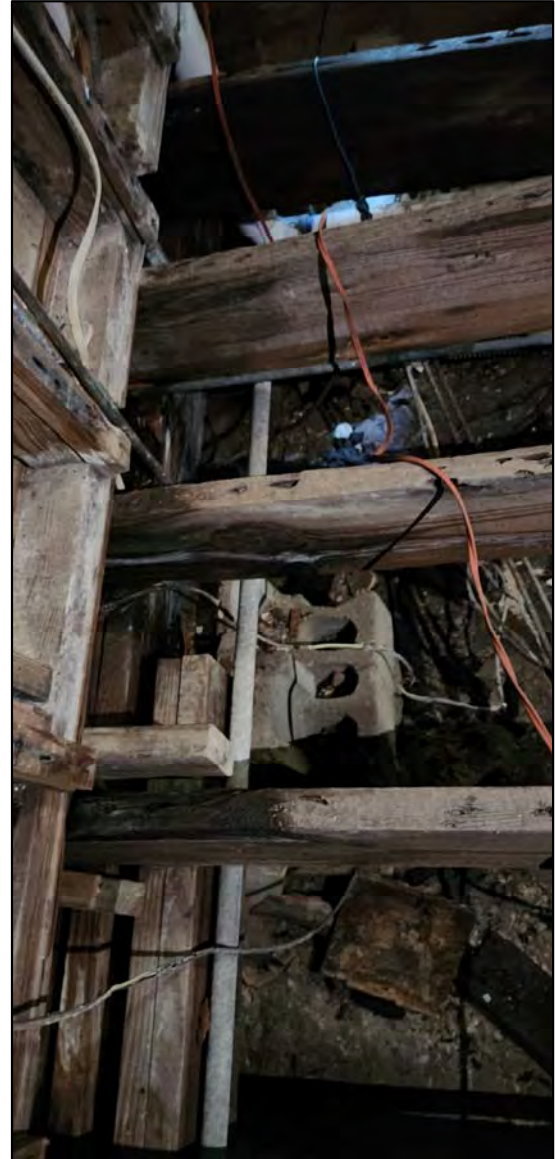
COLLAPSED FLOOR AND DETERIORATED WOOD JOISTS AND WOOD STUDS
