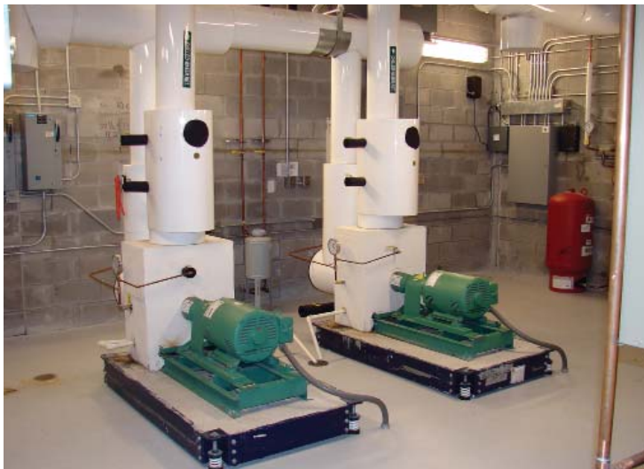
Specialized HVAC/Chiller units to Maintain Precise Humidity in Exhibit Halls
