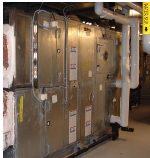
Specialized HVAC/Chiller units to Maintain Precise Humidity in Exhibit Halls
