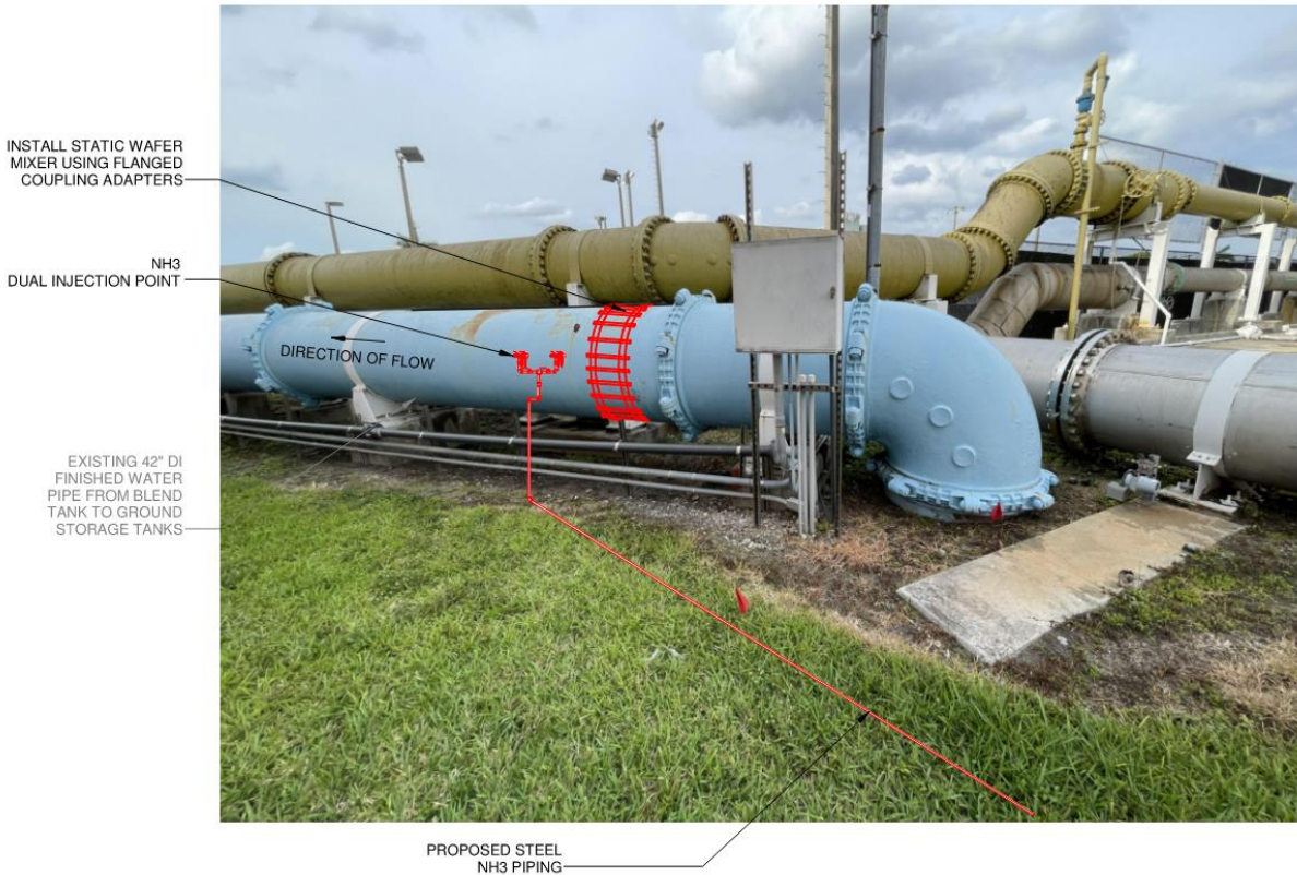
Figure 22: Proposed Ammonia Injection Point
