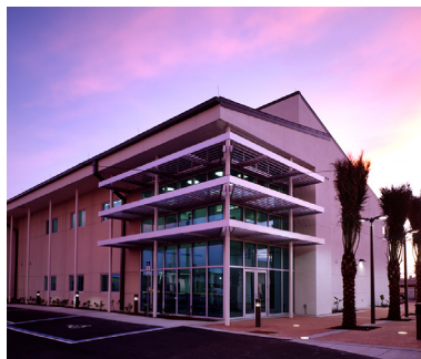
City of Daytona Beach Shores, Public Safety Complex Daytona Beach Shores, FL
