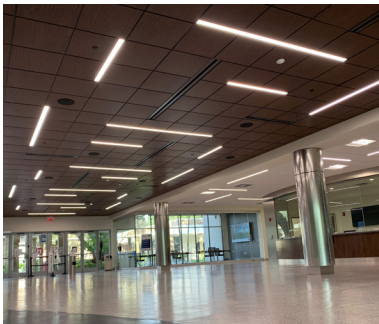
Florida Atlantic University, Student Union Renovations Boca Raton, FL
