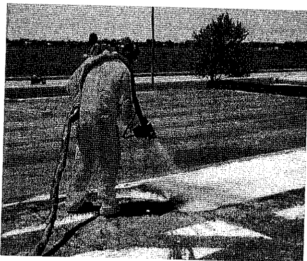
FAST Adhesive is spray-applied to the existing substrate, then insulation boards are set into the adhesive after it develops string/body.
