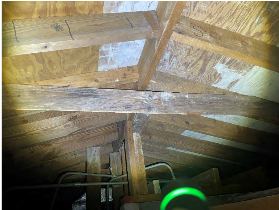
ATTIC AREA ABOVE GARAGE VIEW
