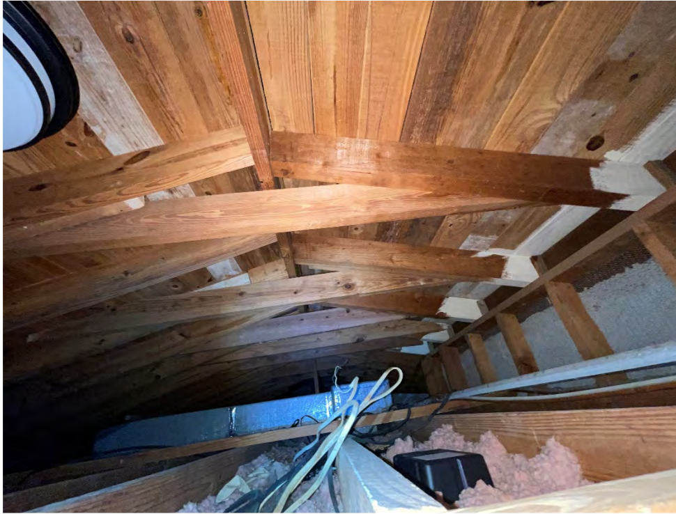
ATTIC AREA ABOVE LIVING AREA VIEW
