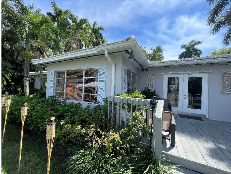
REAR DECK AREA
