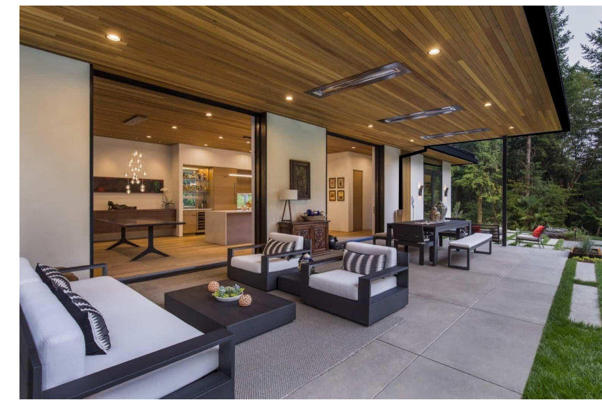
IPE WOOD TO CLAD UNDERSIDE OF MASTER TERRACE BLACK GUTTERS
