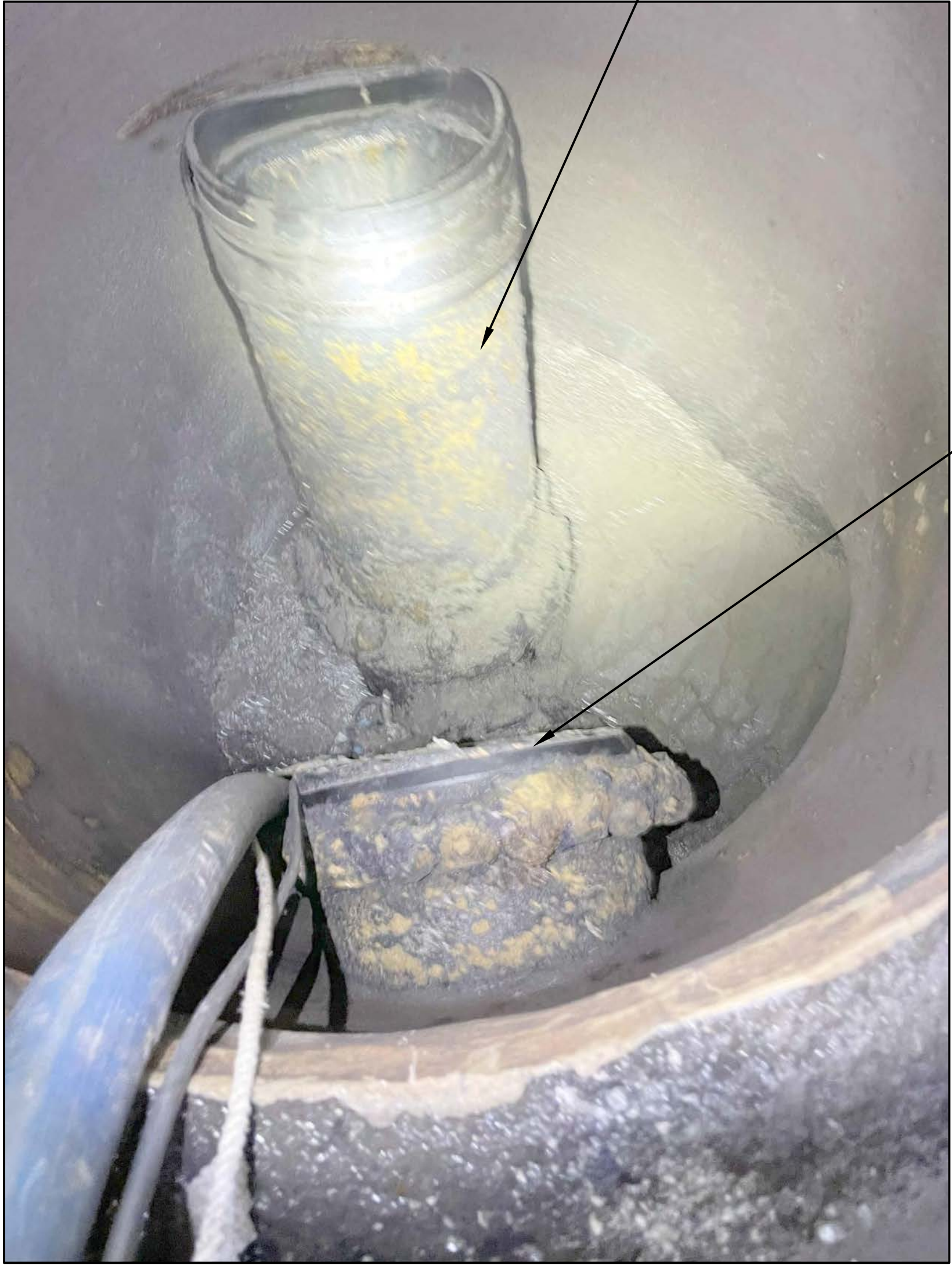
CLARIFIER No. 3 EXISTING 16-INCH RAS LINE REPAIR
