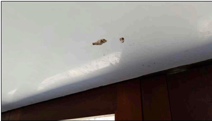
Ceiling damage due to termite
