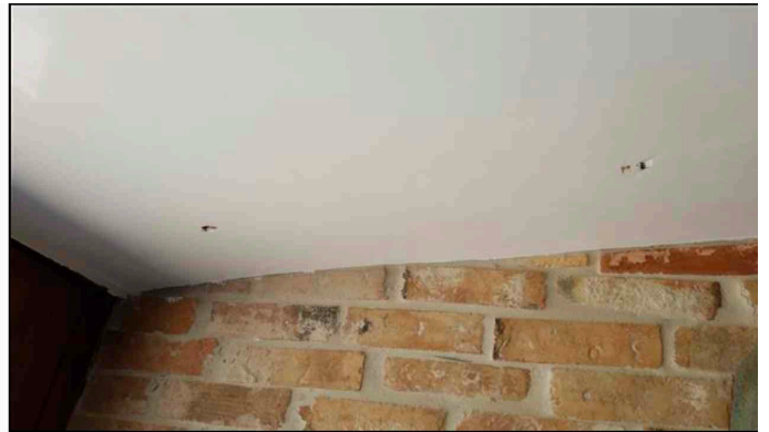
Ceiling damage due to termite
