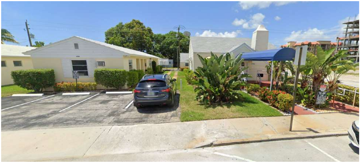
1736 Van Buren Street (east)
