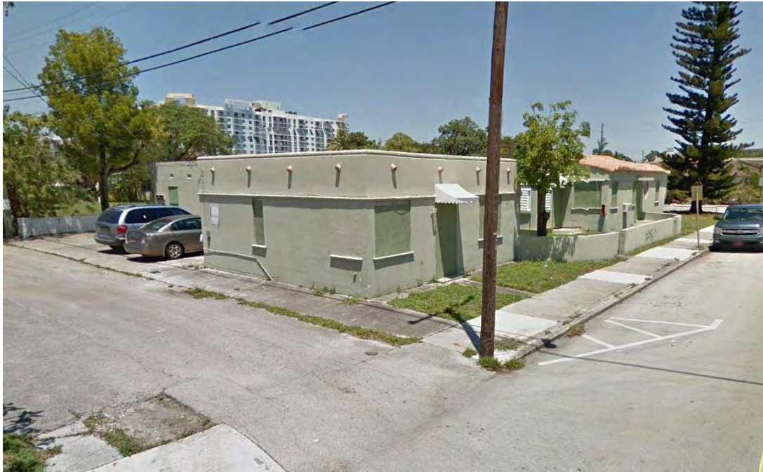
SOUTHEAST CORNER OF SITE
