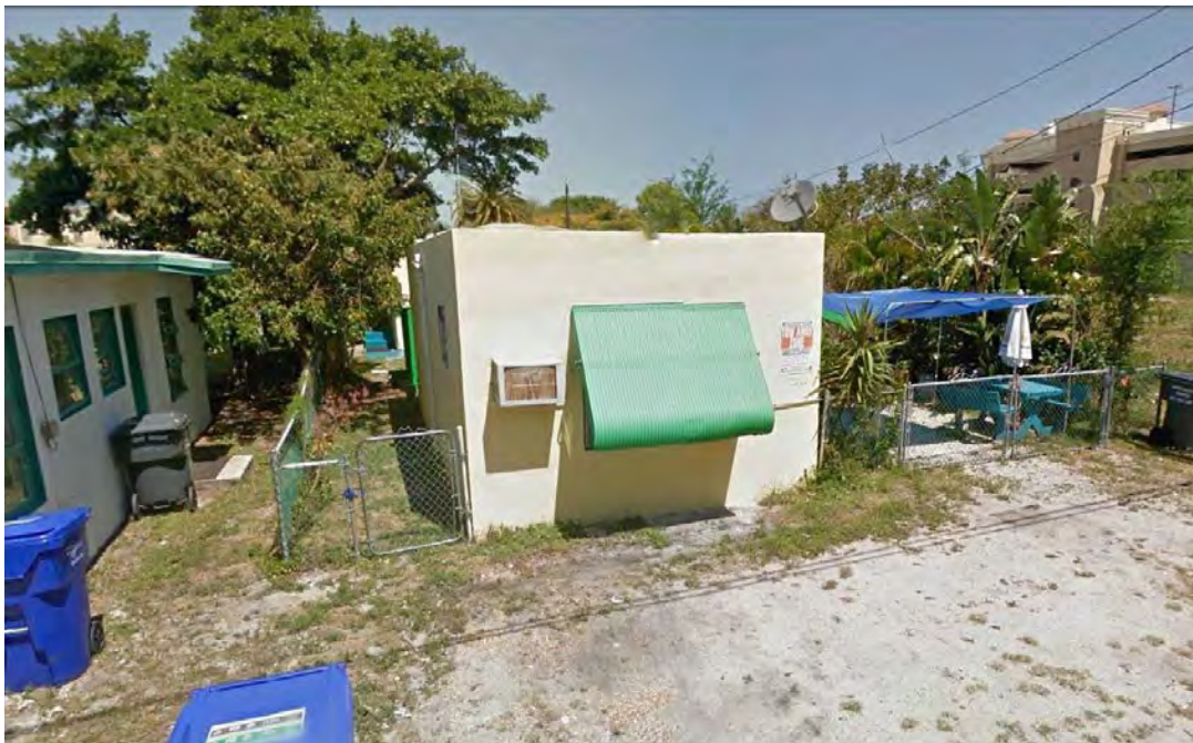
2020 Van Buren (South Façade – Along Jackson Street)
