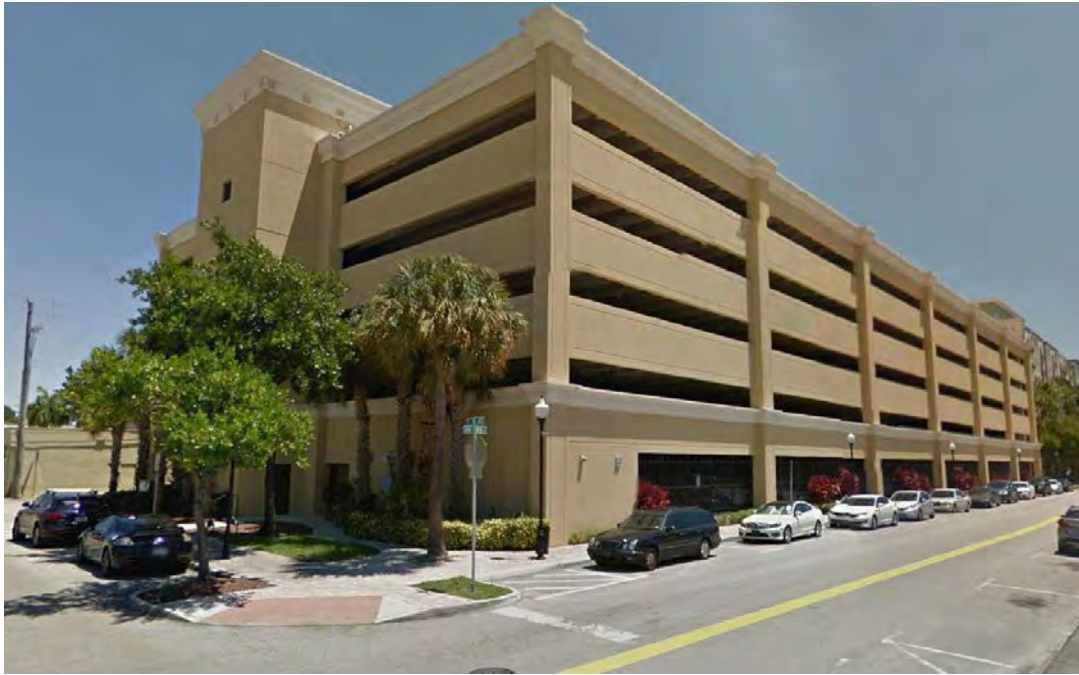
1900 Van Buren (Northeast corner from site)
