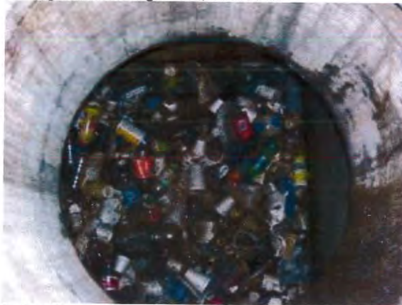
Before Sewer Cleaning
