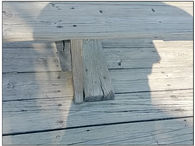
(9) Wood walkway is rotted in various areas. Dock boards are rotted in various area
