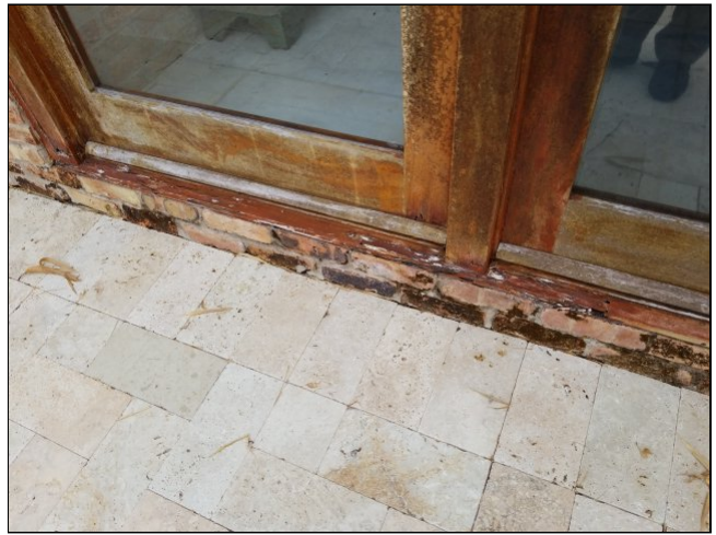
(19) Patio rear door frames has water damage. Recommend replacing bank of doors. $Unknown
