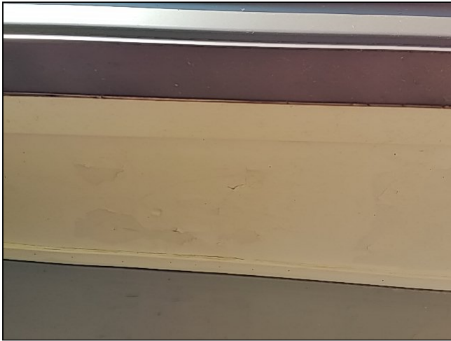
(2) Storage door has water damage, door knob assembly is inoperative and door frame is missing latch plates. Recommend replacing door and frame. $300 to $400
