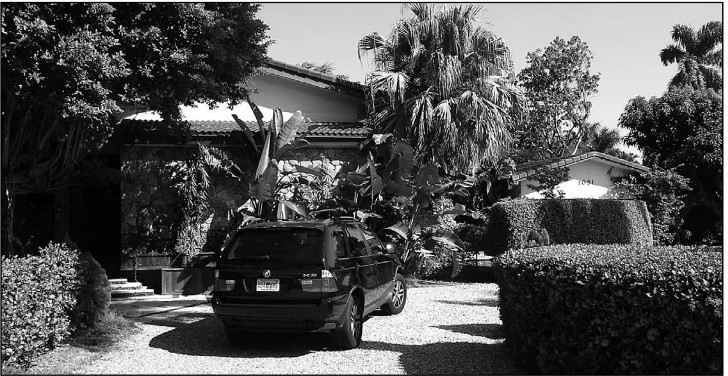
Fig. 22b – Current photo of Ritchie House showing modification inappropriate for the architectural style of the Ritchie House [photo by Louis Friend, 2006]
