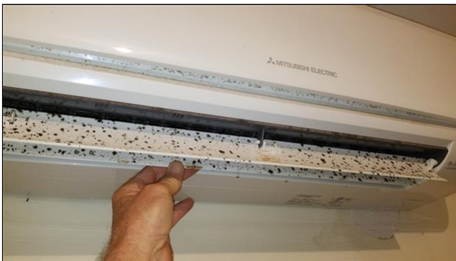
(4) Evidence of mold at interior air handlers. Recommend further evaluation.
