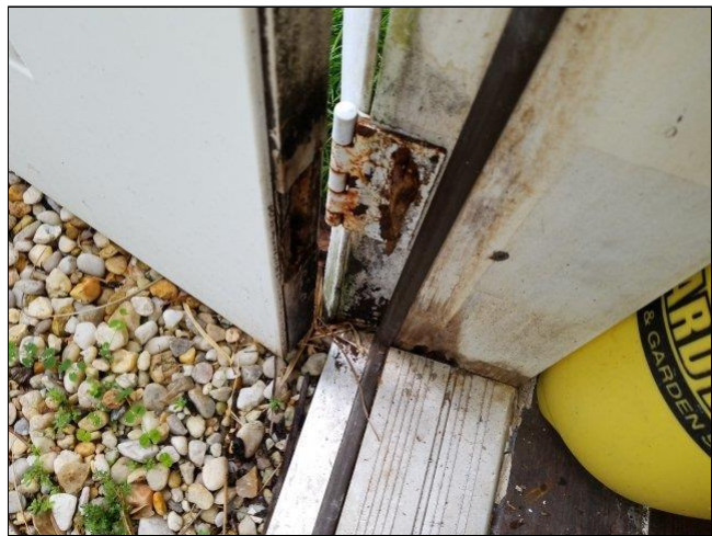
(2) Storage door has water damage, door knob assembly is inoperative and door frame is missing latch plates. Recommend replacing door and frame. $300 to $400
