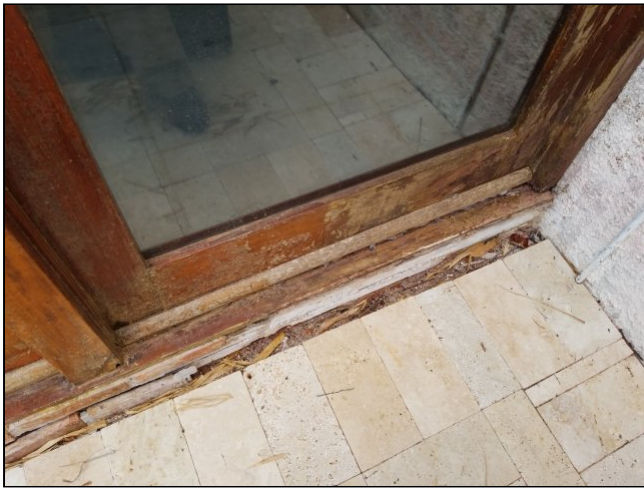
(19) Patio rear door frames has water damage. Recommend replacing bank of doors. $Unknown
