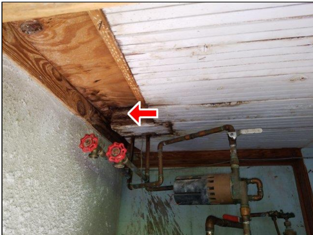
(28) Water closet ceiling sheathing has water stains from a roof leak.
