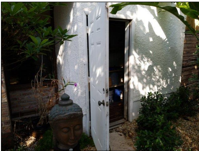
(2) Storage door has water damage, door knob assembly is inoperative and door frame is missing latch plates. Recommend replacing door and frame. $300 to $400
