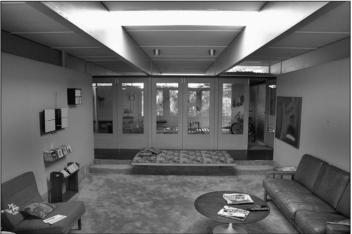
Fig. 18a – Interior of String House, illustrating innovative prefabricated stressed-skin plywood roof joists supporting the large interior span of the living room [photo by Louis Friend, 2006]
