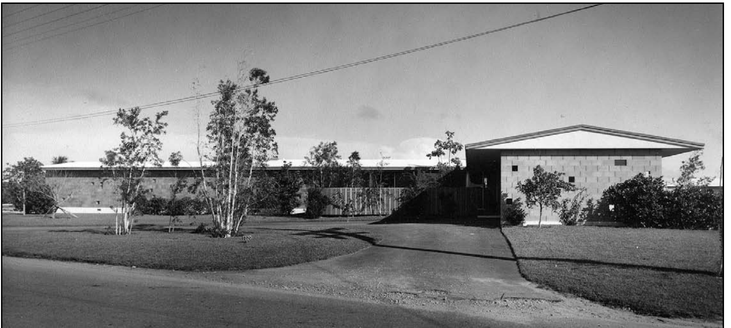
Fig. 19b – Simon House Exterior [photo by Charles Reed, Jr., c. 1960s]
