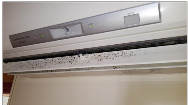
(4) Evidence of mold at interior air handlers. Recommend further evaluation.
