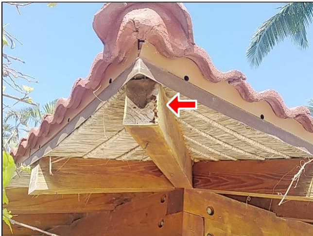
(8) West cabana roof is tilted down, possible subterranean damage. $Unknown
