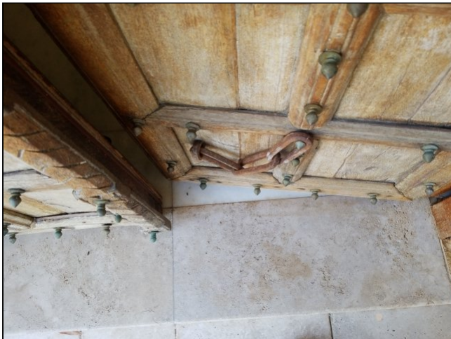
(34) Front door rubs against tile flooring and door does not remain open.
