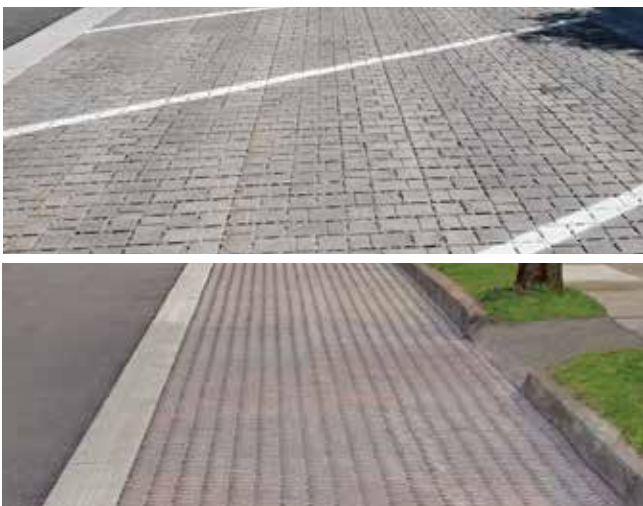
Image 23. Permeable pavers for on street parking examples. (Source: Plant Landscape & Arch Network)
