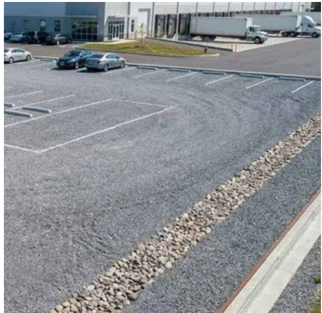
Image 31. Temporary gravel lot example.(Source: basecore)
