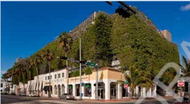
Image 32. Seventh & Collins parking garage.(Source: gateway travel)
