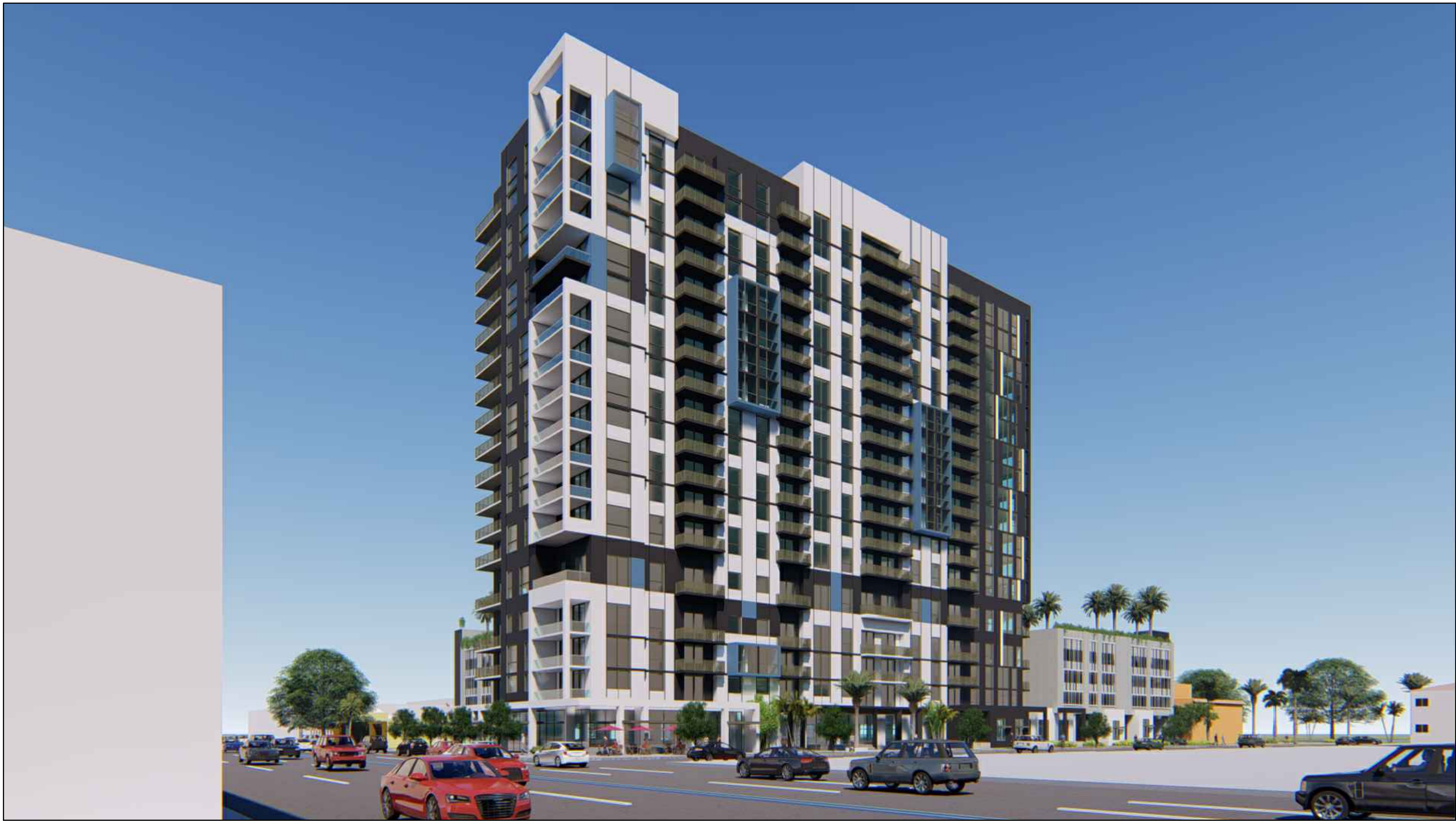
VIEW LOOKING NORTHEAST FROM FEDERAL HWY
