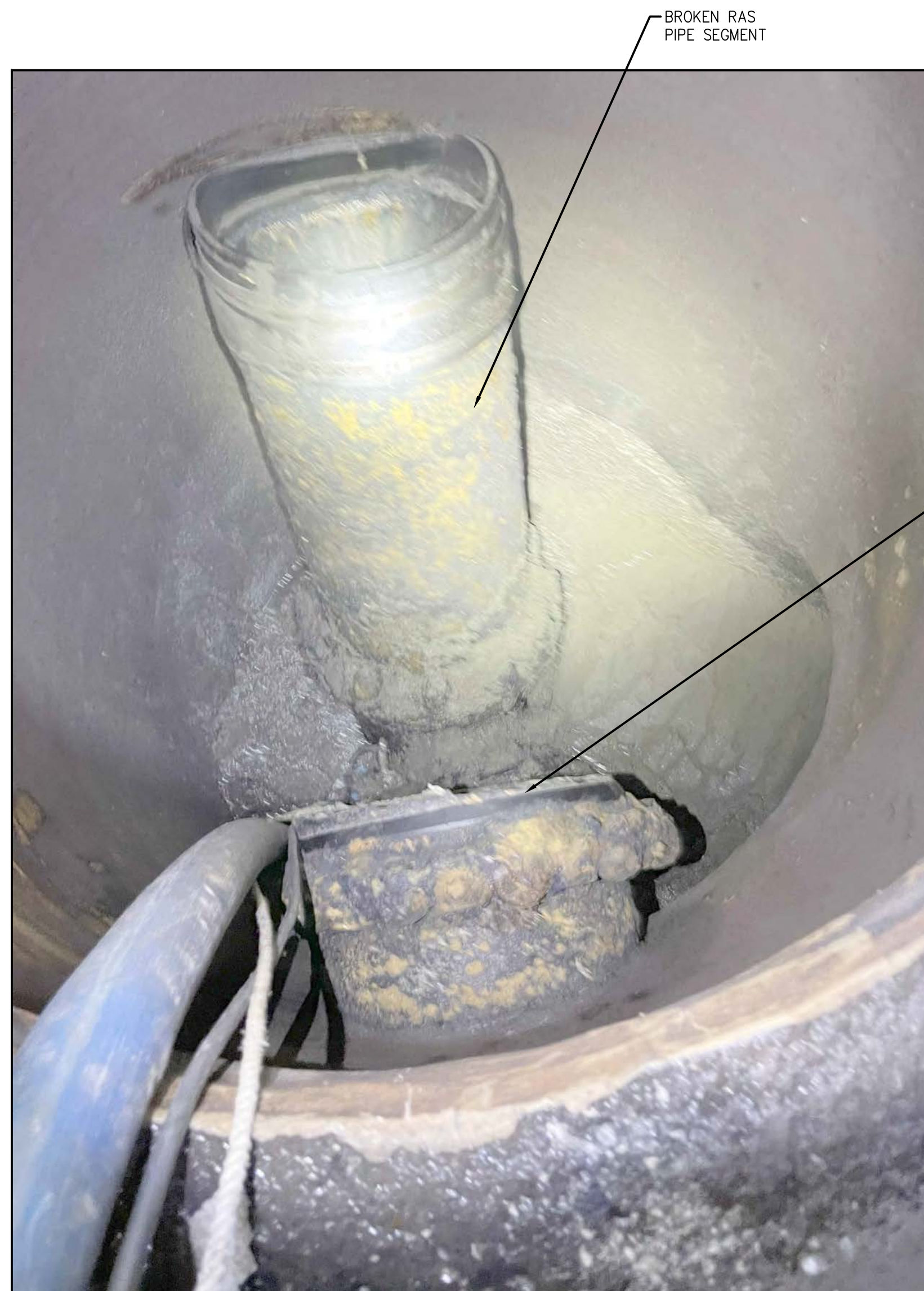
CLARIFIER No. 3 EXISTING 16-INCH RAS LINE REPAIR
