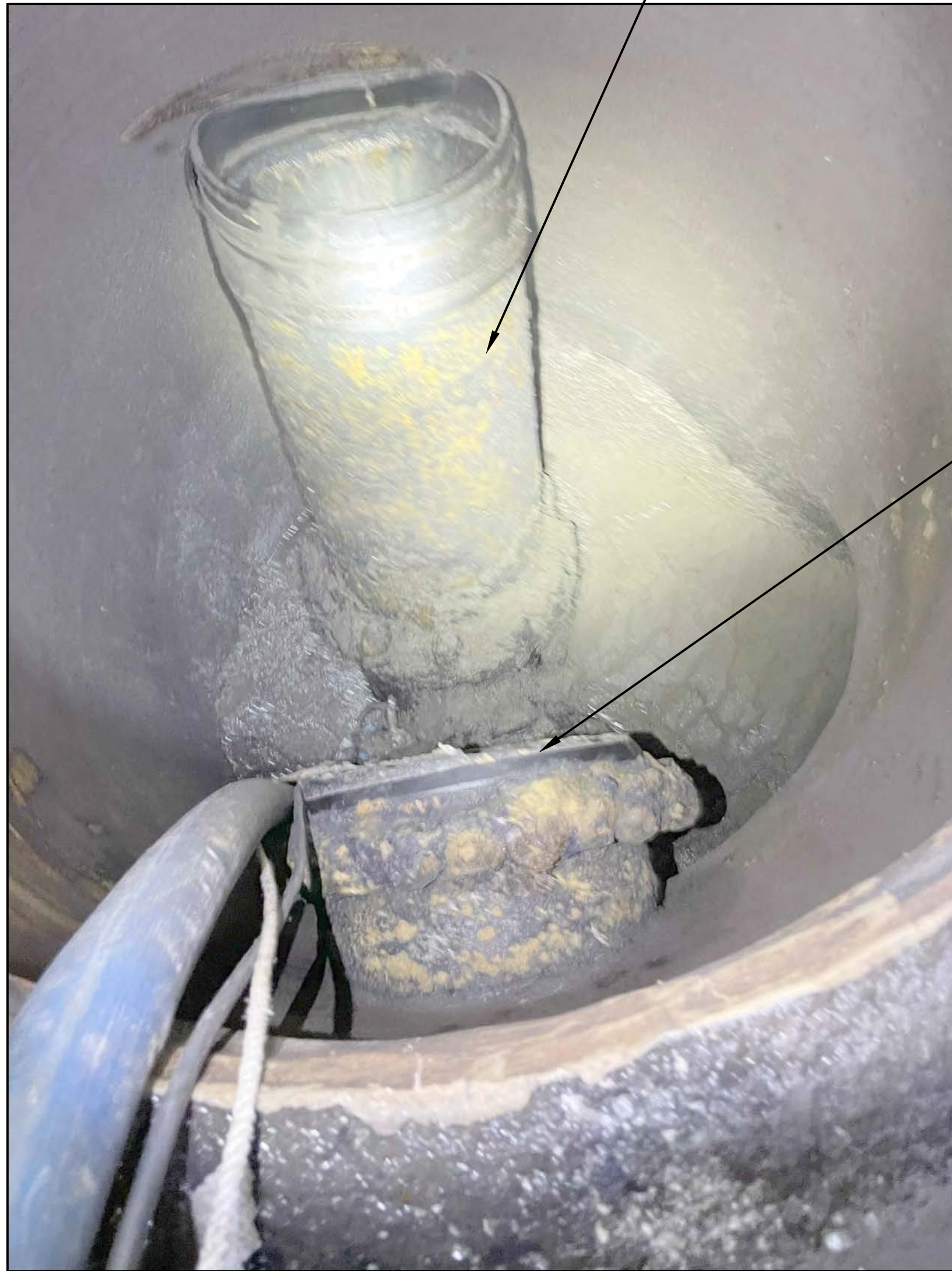
CLARIFIER No. 3 EXISTING 16-INCH RAS LINE REPAIR
