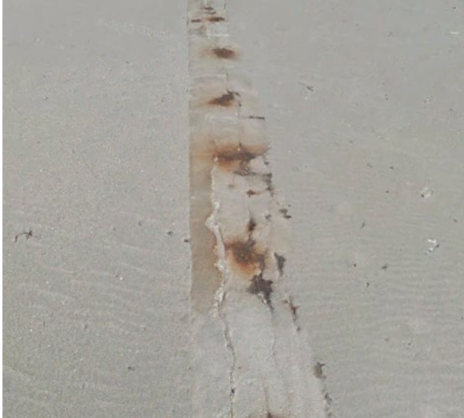
Figure 4. Cracking and rust stains observed on the northern portion of the seawall.
