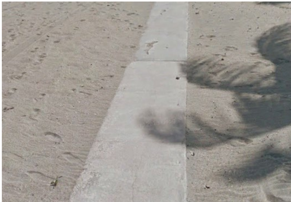
Figure 5. Cap on seawall in front of southerly adjoining property.
