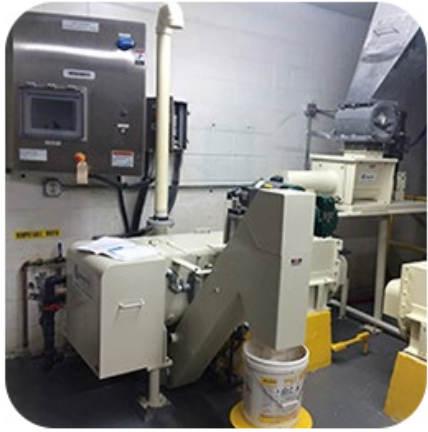
Nebraska City WWTP, NE
