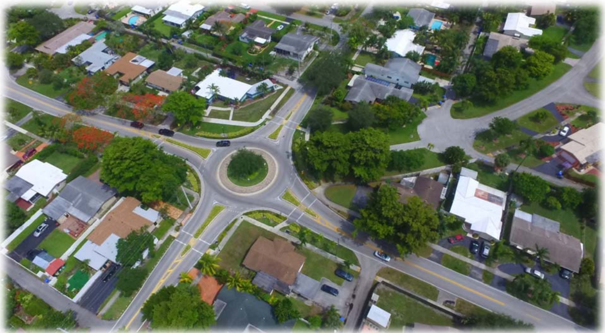
Figure 8 Taft Street and 40th Avenue Roundabout
