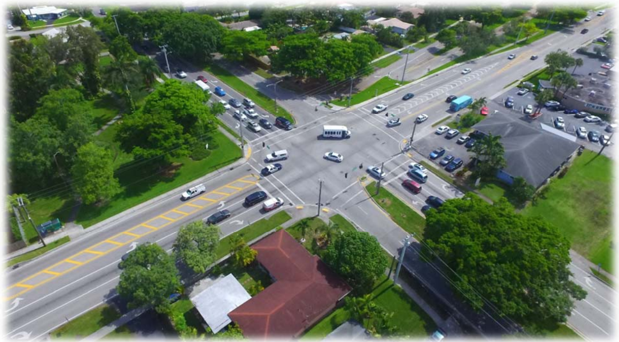
Figure 11 Johnson Street and Park Road intersection
