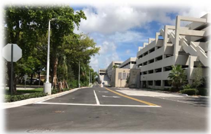
Figure 3 New parking garage driveway for Memorial Regional Hospital at Johnson Street
