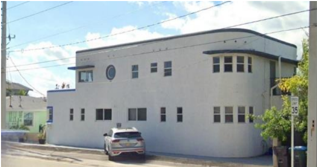
2200 N. Ocean Drive (south of subject site)
