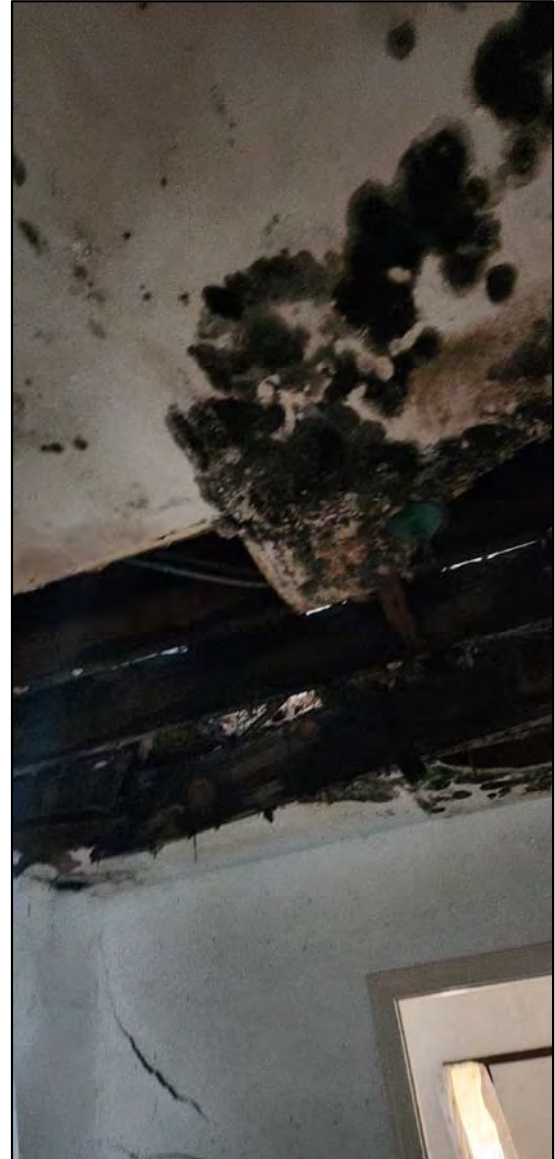
COLLAPSE OF INTERIOR OF FIRST FLOOR
