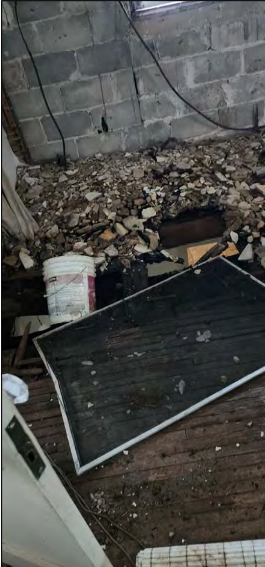
COLLAPSE OF FIRST FLOOR
