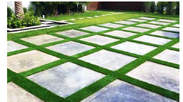
Concrete slabs with turf at Driveway
