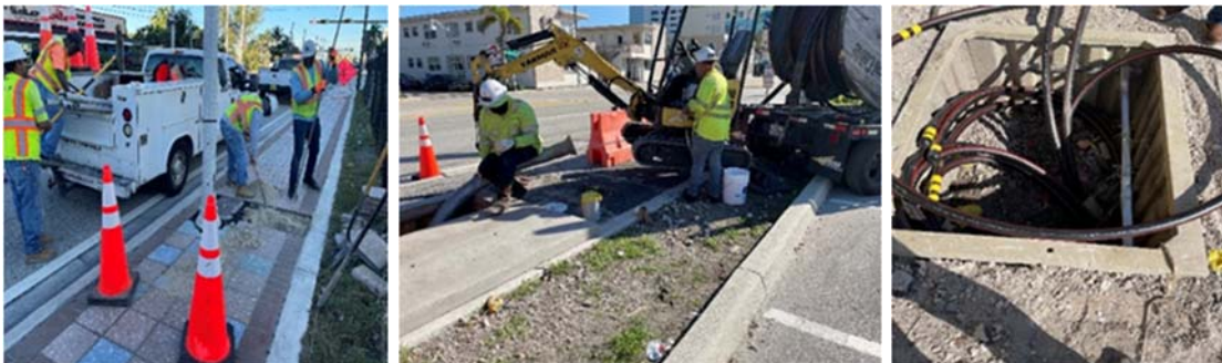
Pulling underground primary cable and electrical wiring at various locations.
