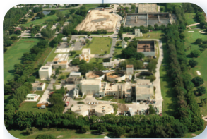
City of Hollywood SRWWTP Upgrades $26.21 million
