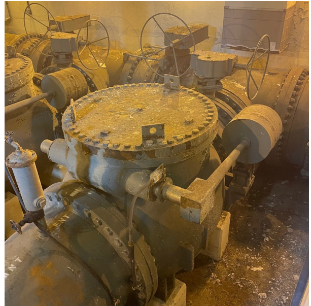
General view of the mechanical equipment for the pump discharge including a swing check valve.
