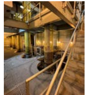
Extended shafts from existing IPS pumps, with motors mounted on the upper floor.
