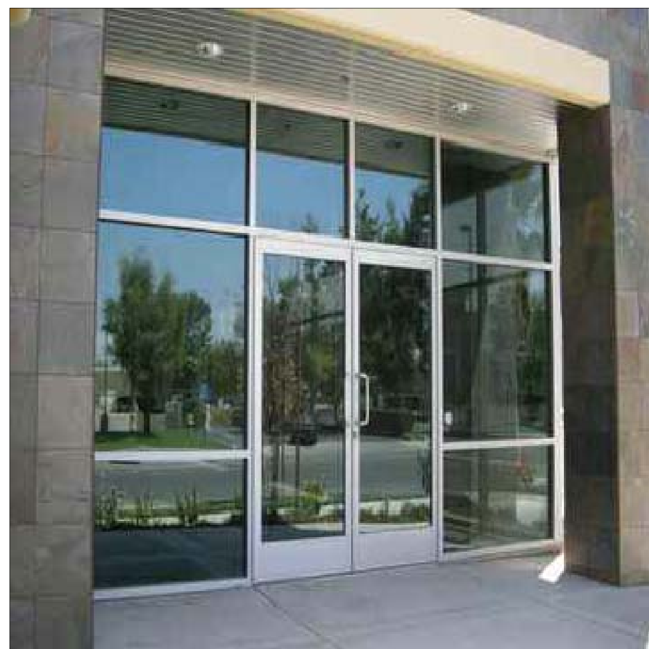
ENTRY DOOR AND FRAMING STYLE
