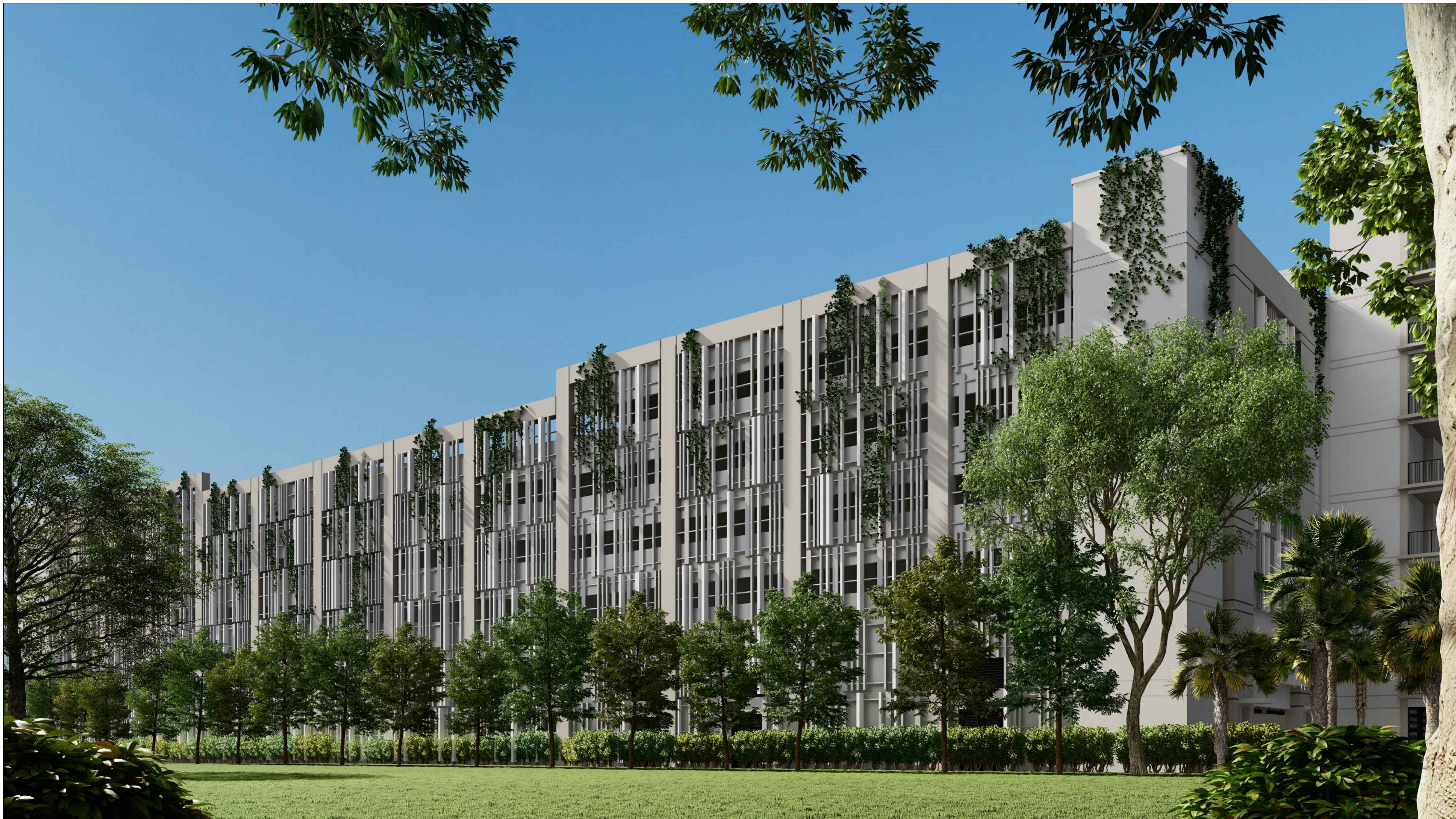
PARKING GARAGE SOUTH - WEST ELEVATION VIEW
