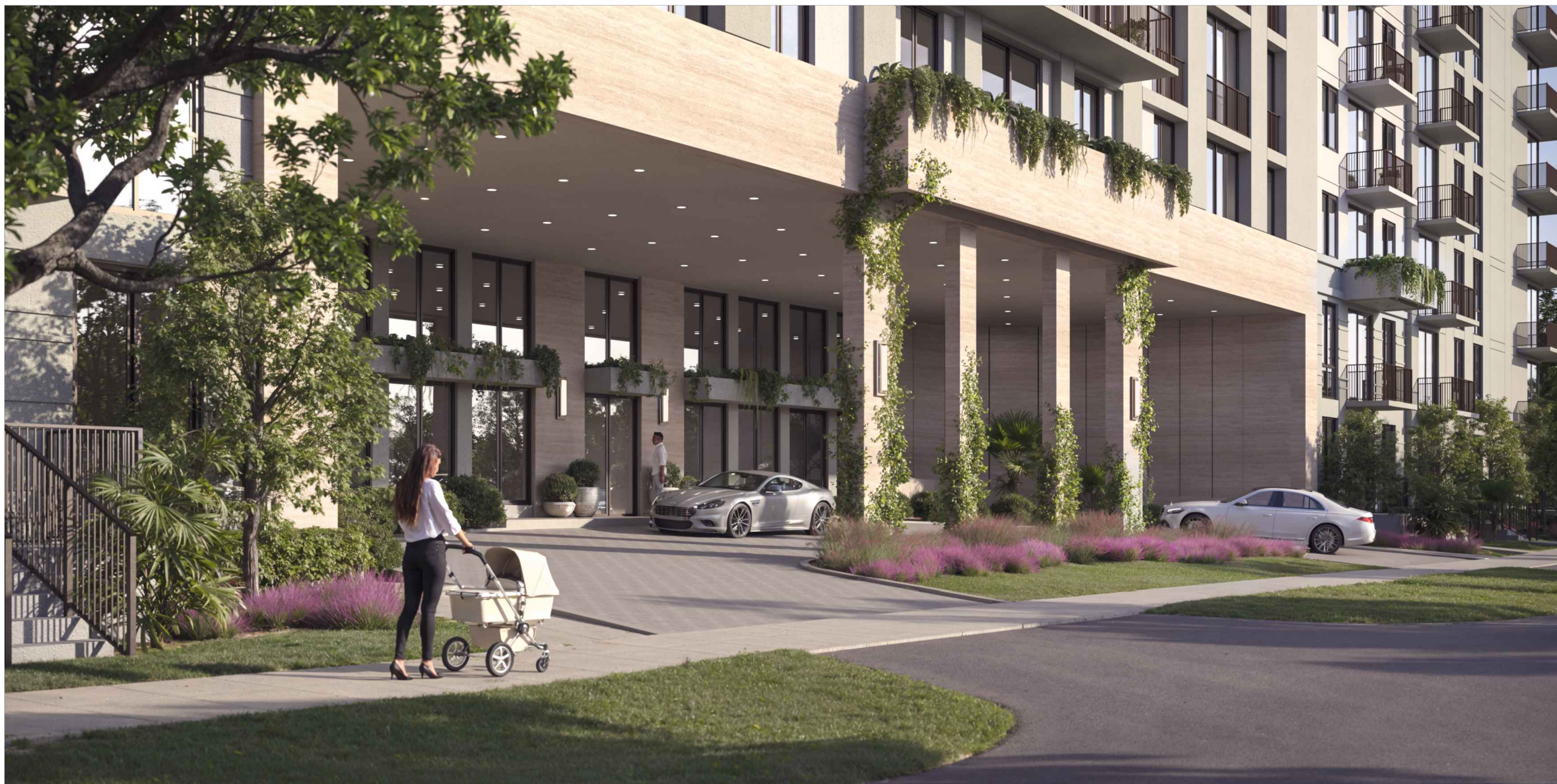
VIEW OF THE EAST DROP-OFF AREA VIEW FROM DAVIE ROAD (N 58th AVE)
