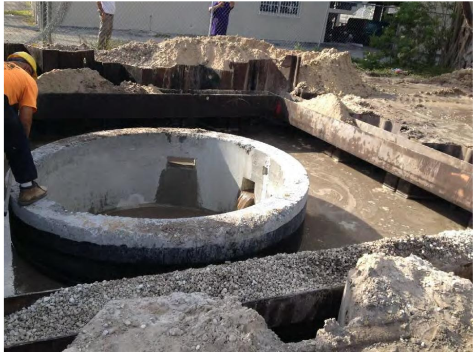
Opa-locka sewer pump station rehabilitation.
