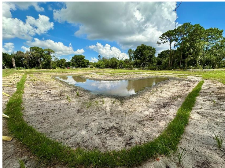
Ancient Oaks stormwater pond shortly after landscape installation.
