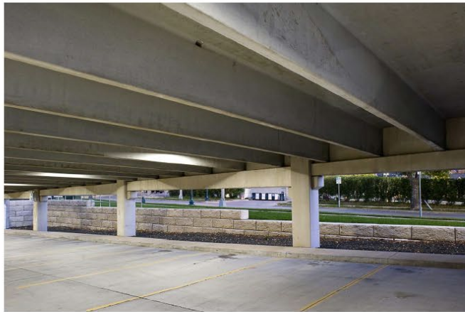
EXPOSED PRECAST CONCRETE STRUCTURE AT GARAGE LEVEL
