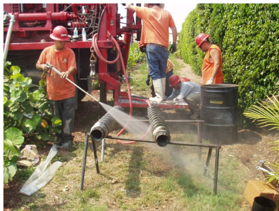
URS drilling crew in operation at the former Hollywood Incinerator Ash Landfill site on 1600 South Park Road
