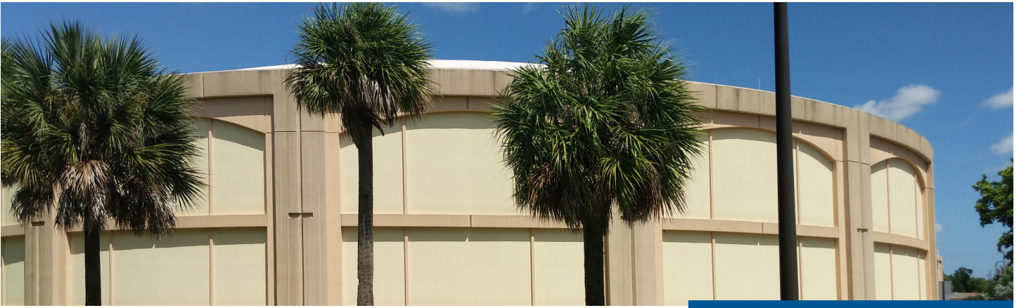
West Hollywood Pumping & Storage Facility
