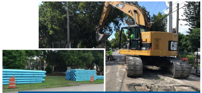
16-Inch DIP water transmission main construction along N. 19 Avenue in the City of Hollywood
