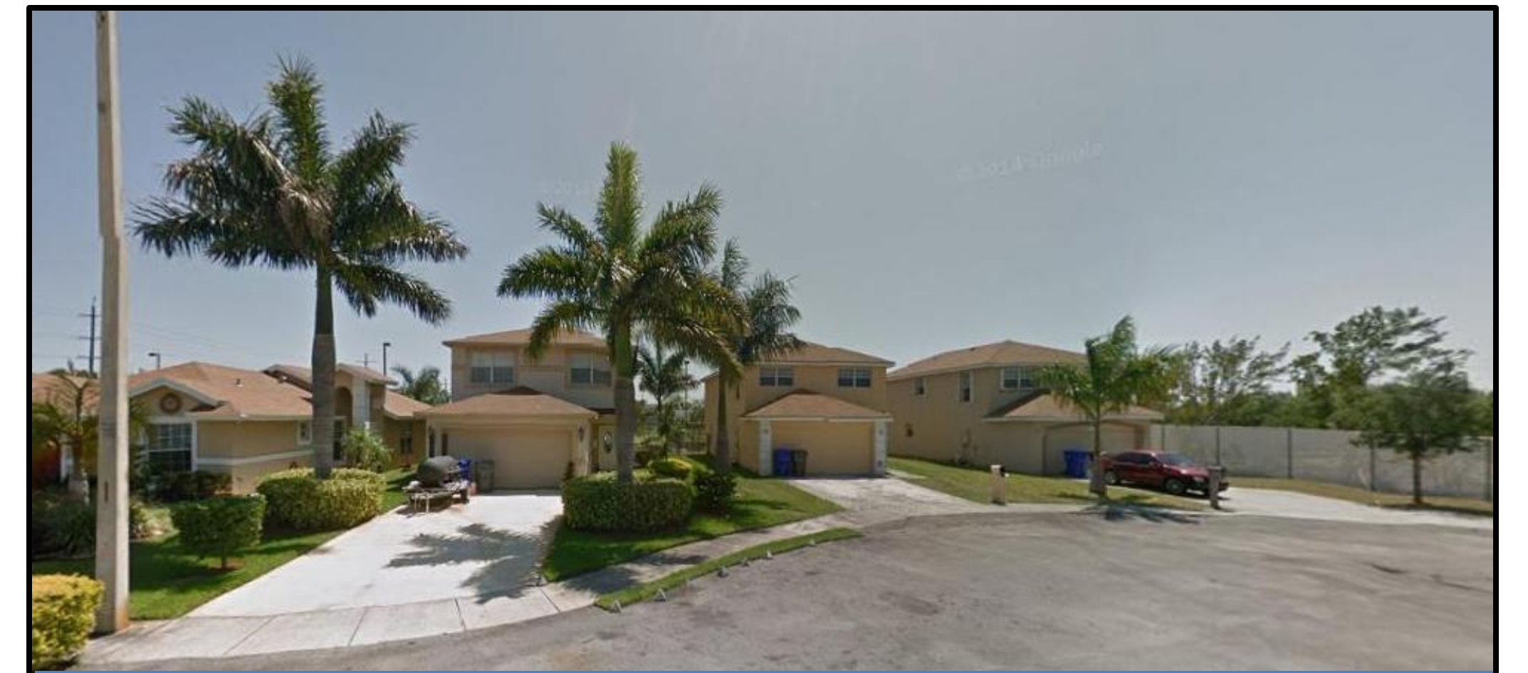
South View - West
