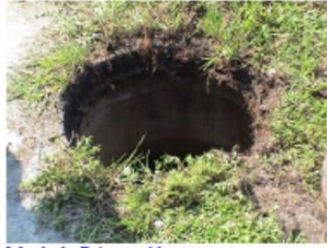
Manhole Prior to Abatement
