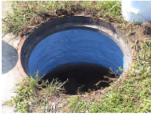
Manhole Following Abatement
