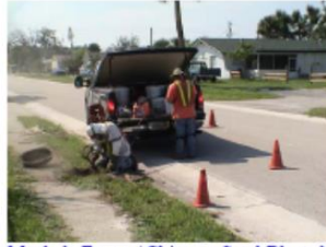
Manhole Frame / Chimney Sand-Blasted
