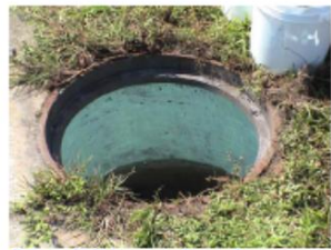
Frame & Chimney - Prime Coat
