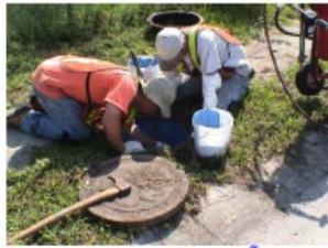
Frame & Chimney - Elastaseal® Coat
