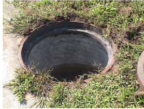
Manhole Interior Following Sand-blasting
