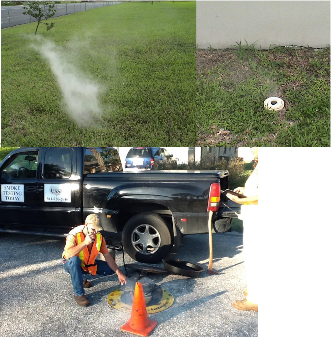
Figure 11 a, b, c Smoke Testing
