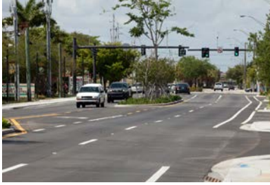
Dr. Martin Luther King, Jr. Boulevard Water main & Streetscape Improvements
