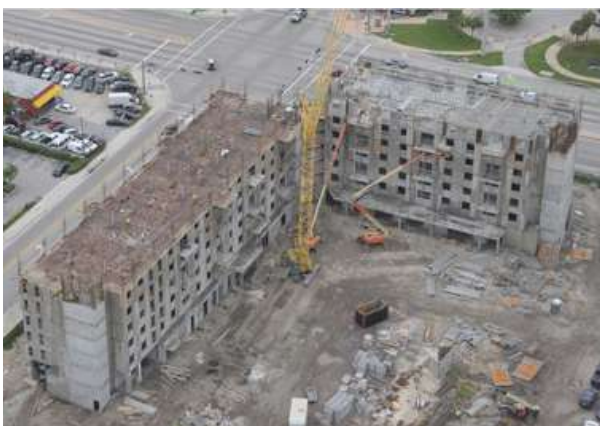
Pinnacle 441 Phase 1 Under Construction
