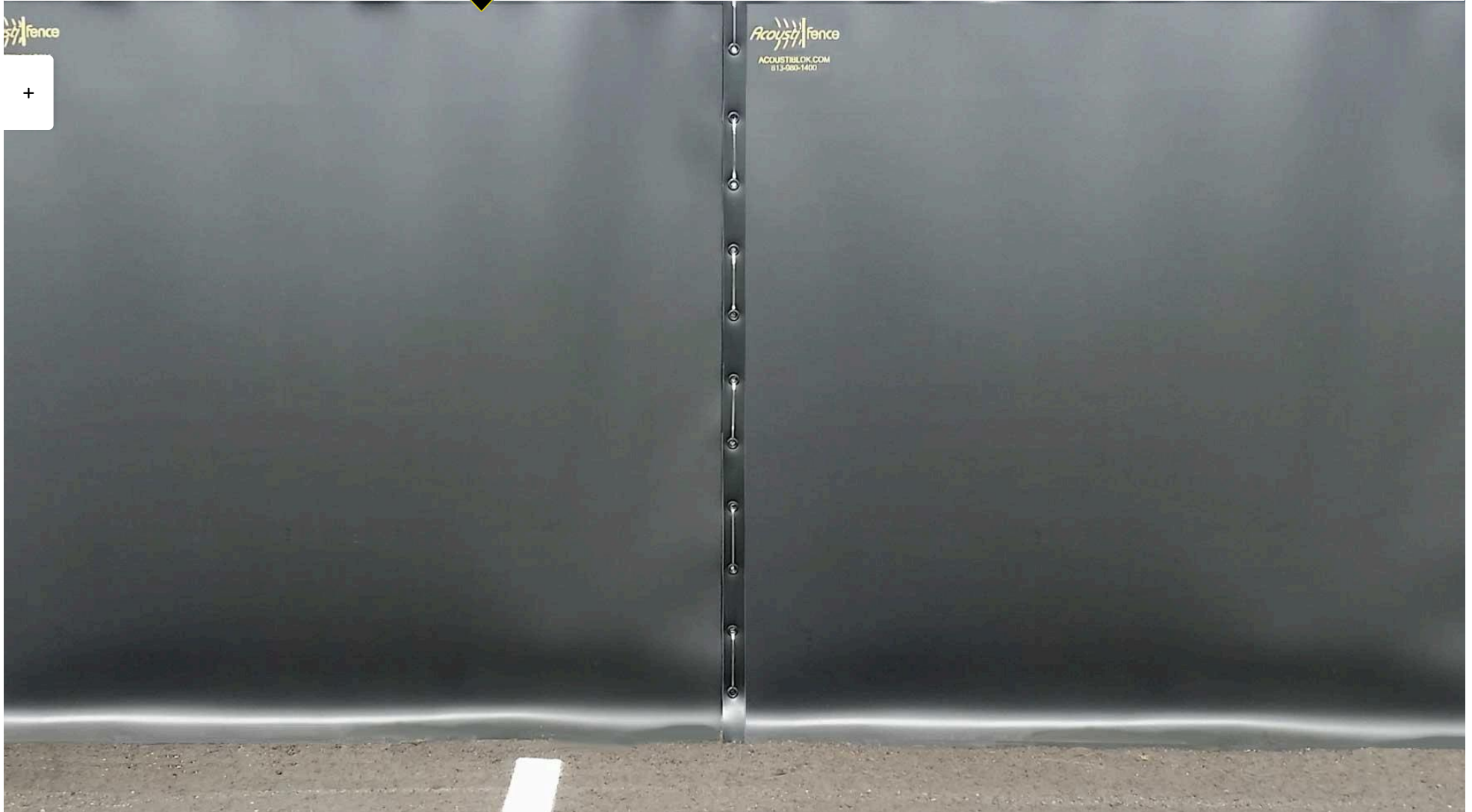
Acoustifence Installed with Stainless Steel Ties
