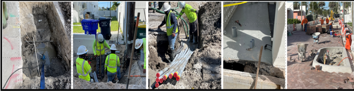
Horizontal Directional Drilling at A1A for electrical infrastructure and undergrounding work.
