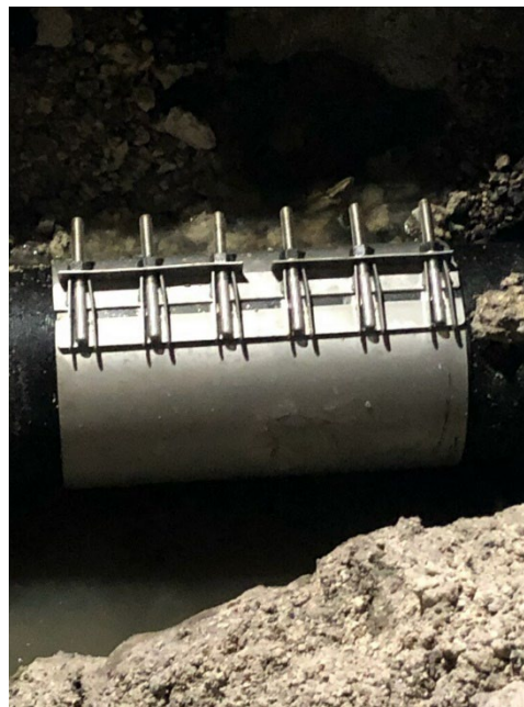
Section of Pipe Restored with a Clamp
