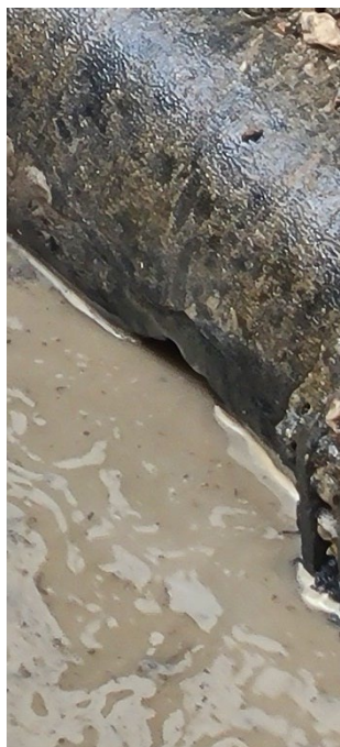
Wastewater Leaking from a Hole in the Pipe
