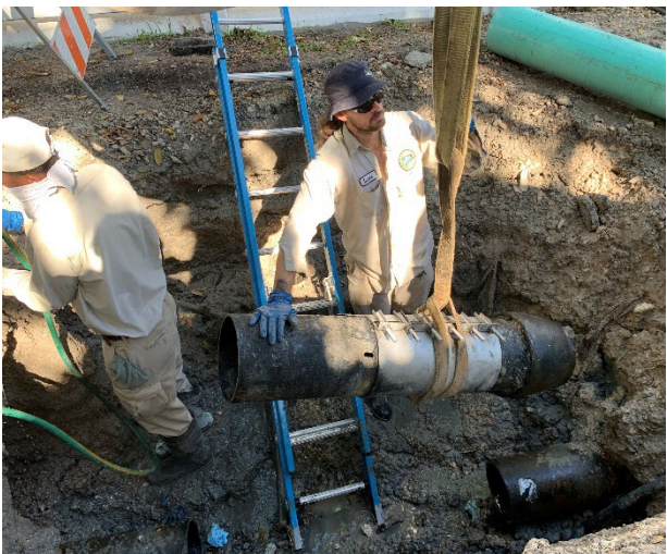
Section of Pipe Restored with a Clamp
