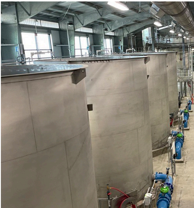
Pellet softening system at the South Adams County, CO, Water and Sanitation District Facility.
