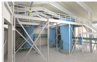
New pellet softening system will reduce the need to handle lime.
