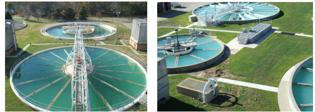
Lime softening basins operating in conjunction with membrane treatment at Olathe, KS, 37-mgd WTP.
