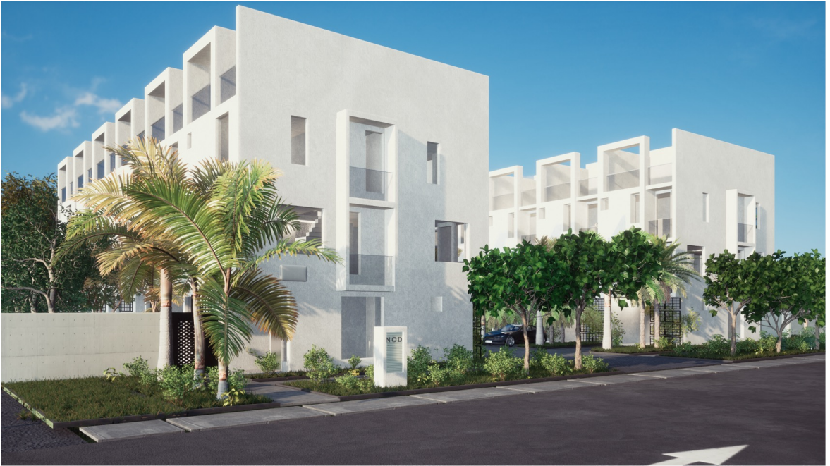
View from Johnson St
