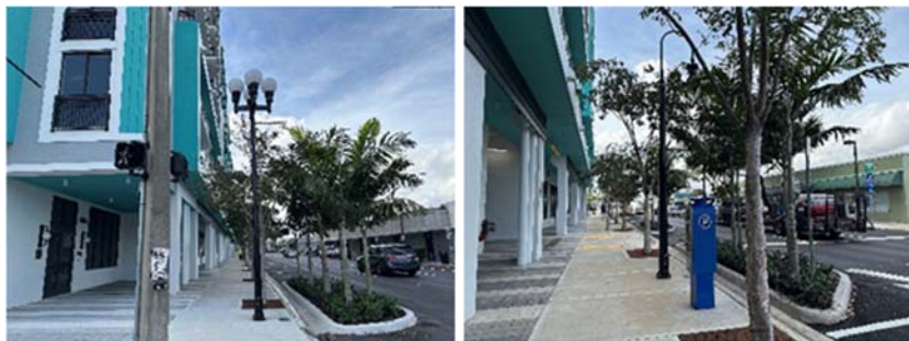
Installation of new light poles and fixtures
