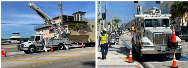
AT&T connection and overhead wire removal
