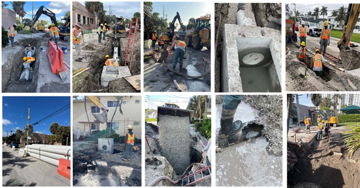
Excavation, trenching, existing conditions evaluation, compaction, and structures installation – Jan. 2025
