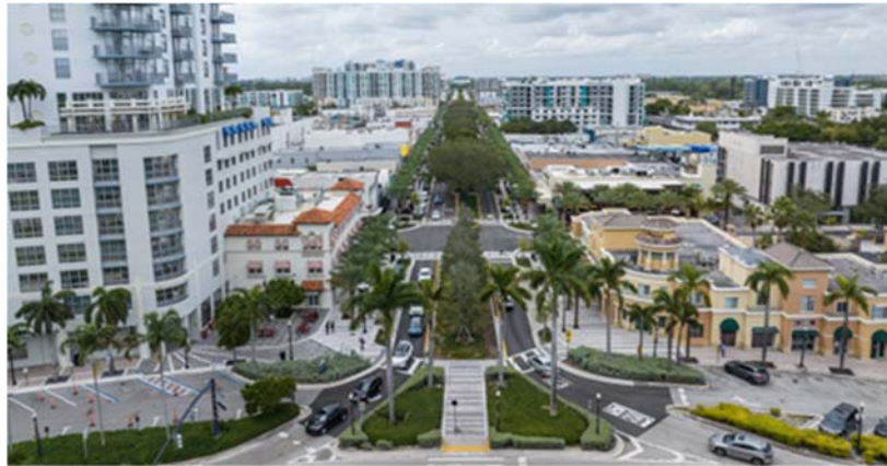
Aerial view of completed streetscape
