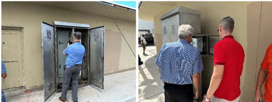
Assessment of electrical and irrigation systems
