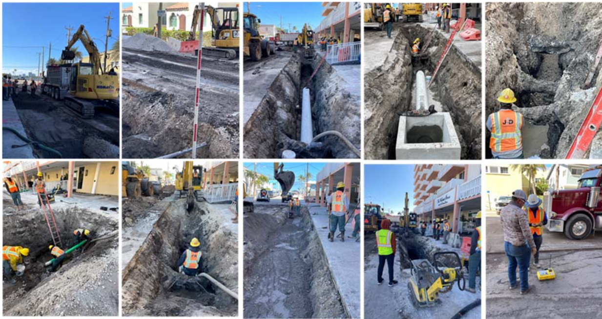
Excavation, trenching, existing conditions evaluation, compaction, and structures installation
