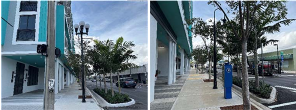
Installation of new light poles and fixtures
