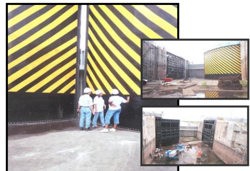
S-310 Navigation Lock Rehabilitation
