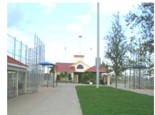
Spanish River Athletic Facility
