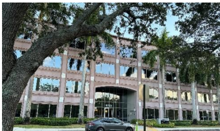
Vanderbilt Office Property 25 Year Inspection
