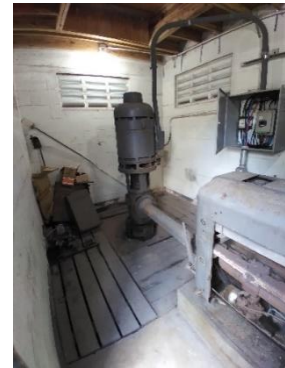
Hook Square Pump Station Rehabilitation
