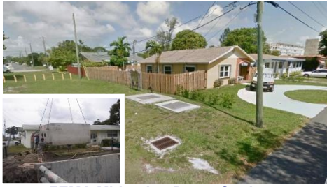
FEMA Mitigation Pump Station Hallandale Beach, Florida
