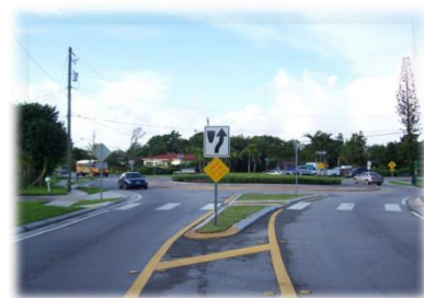
NW 146 th St/N. Miami Avenue/S. River Drive Roundabout
