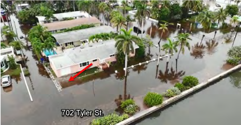
Figure A-4 - Drone Footage at 702 Tyler St.
