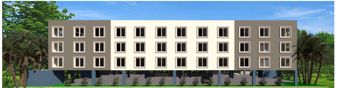
BACK OF BUILDING
