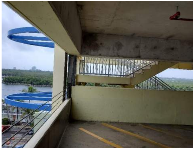
Figure 5. Garfield Street Garage
