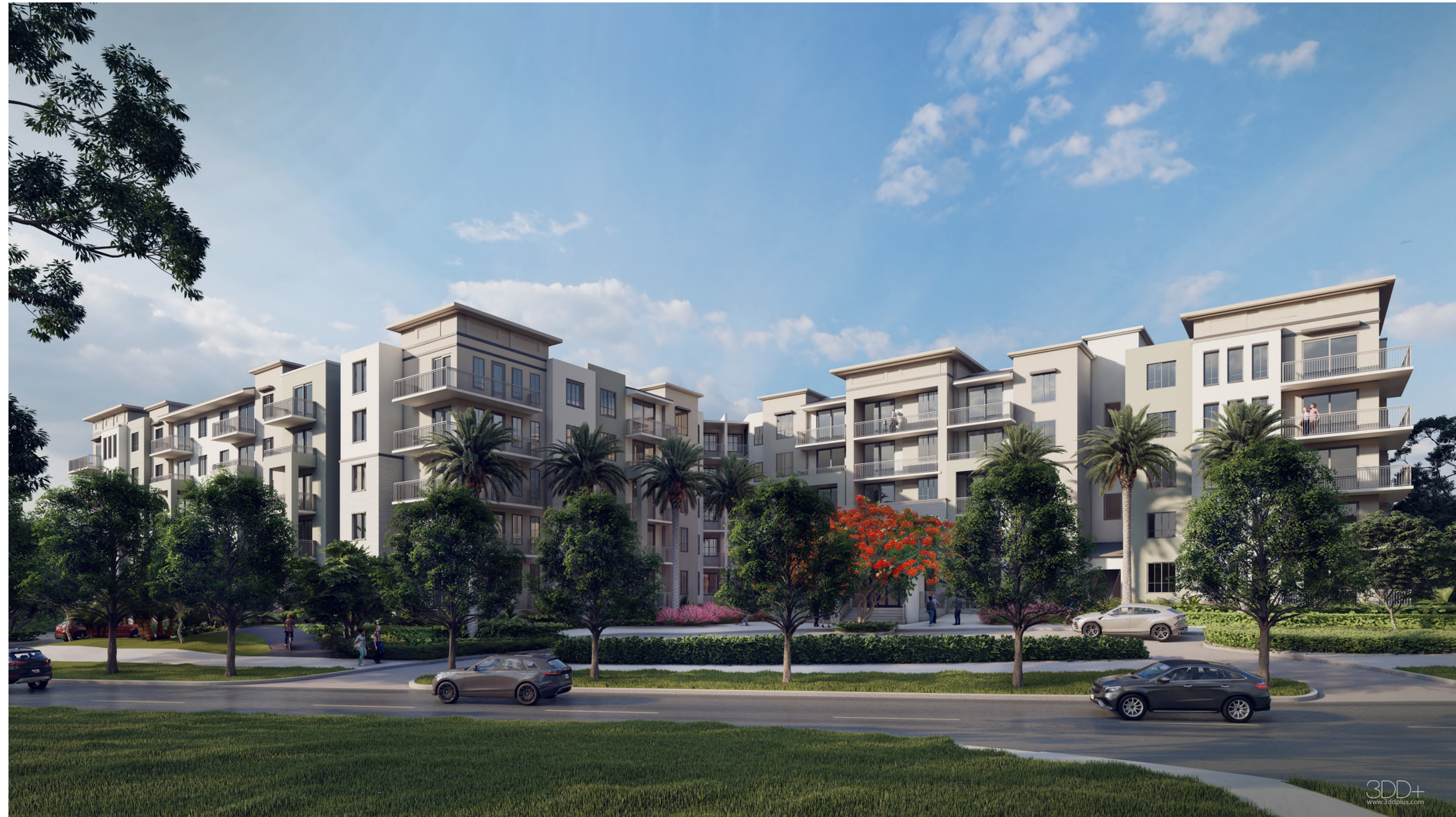
VIEW FROM HILLCREST DRIVE
