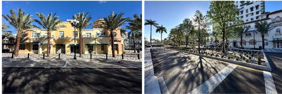
Phase 3 & 4 Substantially Completed
