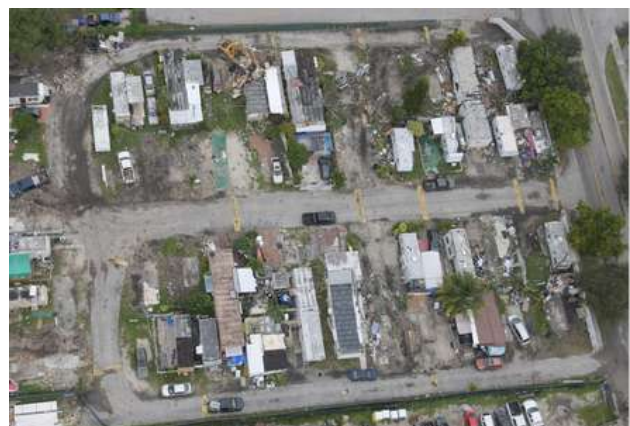
Pinnacle 441 Phase 2 Site (Trailer Park)
