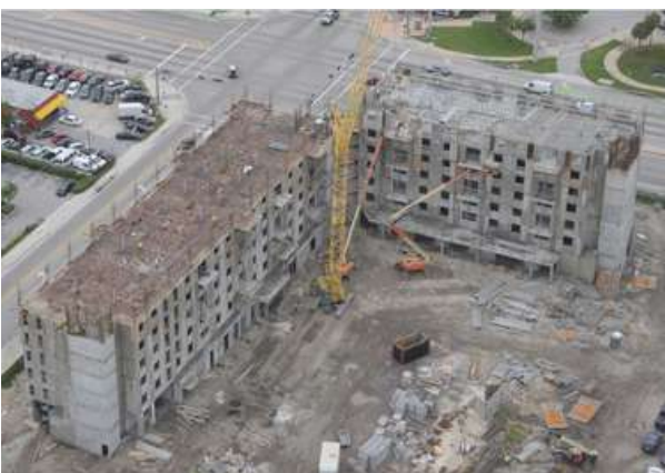
Pinnacle 441 Phase 1 Under Construction
