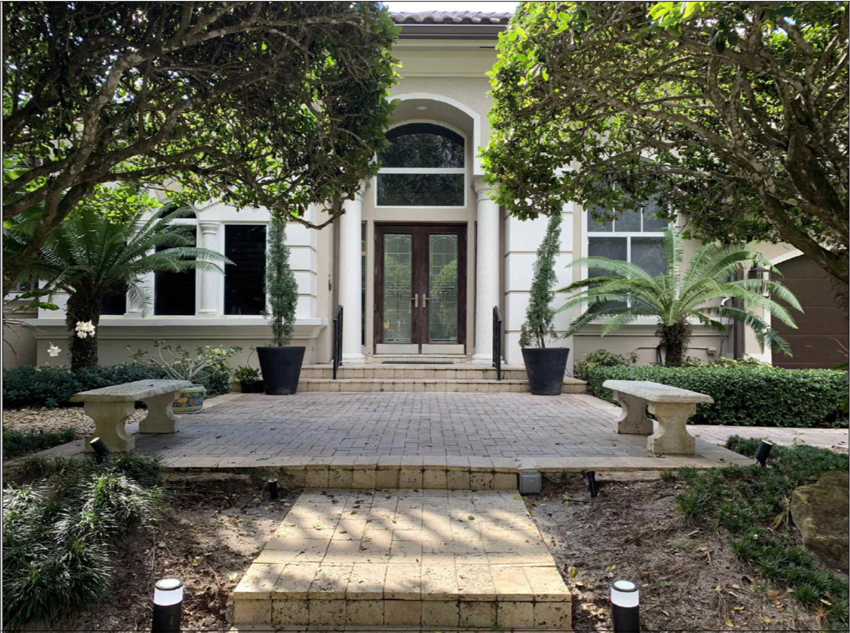
5441 ESTATE OAK CIR. EXIST. FRONT DOOR
