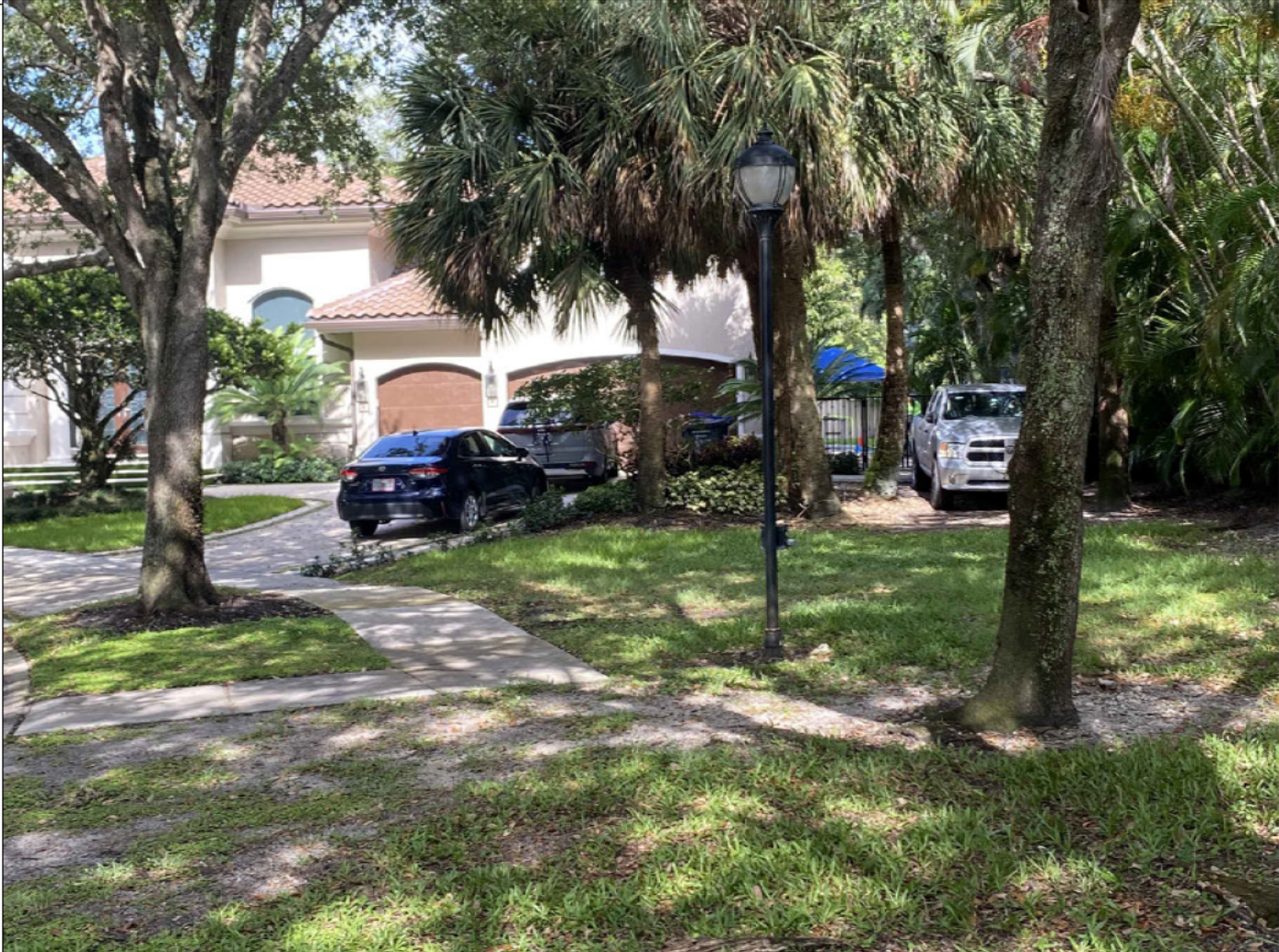
NORTH SIDE EXISTING WALL AND LANDSCAPING
