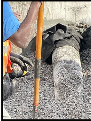
Backfill storm pipe
