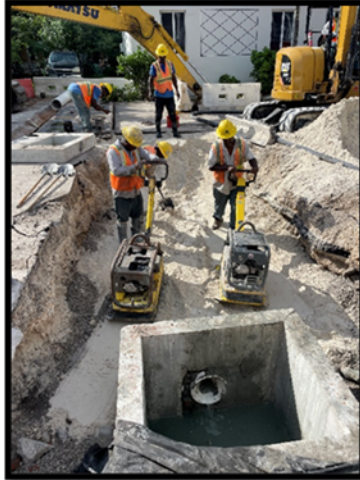
Storm inlet structure
