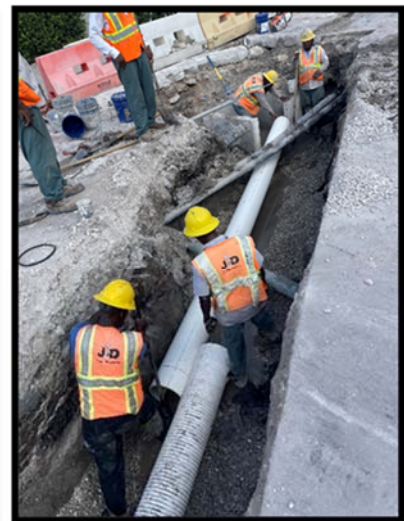
Storm drain pipe installation
