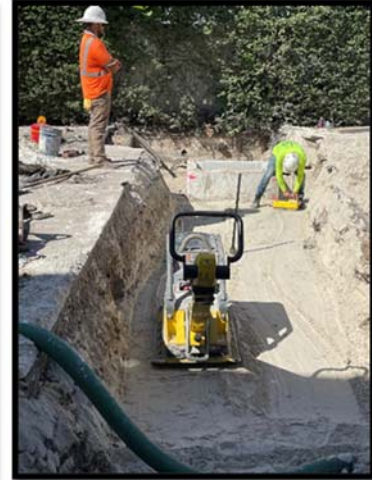
Compaction and testing
